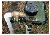
lid (some backflow preventers are above ground). Once you find it, remove the lid and find the two levers on either end of the device. Rotate one or both of them one-quarter turn (or 90 degrees) so that the handle of the lever is perpendicular with the water pipe. See how in our irrigation shut-off video – <u>https://www.youtube.com/watch?v=9wAyEo-01GLM&feature=youtu.be</u>.
